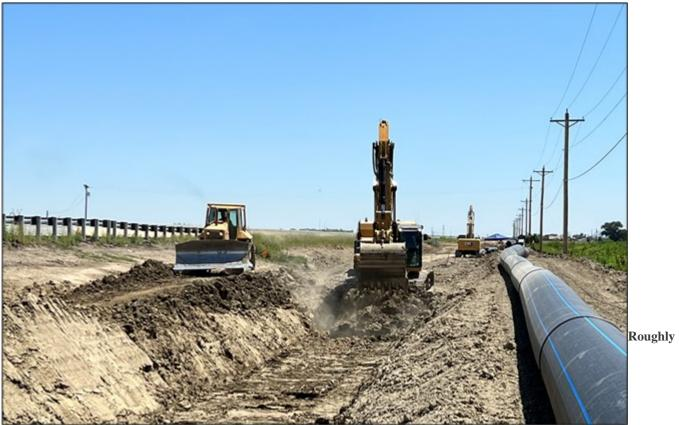
1,000 linear feet of 30-inch diameter HDPE pipe has been welded for the Arkansas Valley Conduit trunk line. It will be placed in a trench 9 feet deep, which is being excavated by heavy equipment on Thursday, July 27, 2023. (Photo by Southeastern Colorado Water Conservancy District.
