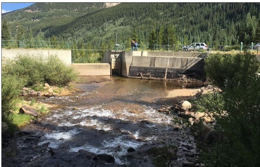
Part of the Fryingpan-Arkansas Project Collection System near the Boustead Tunnel.
