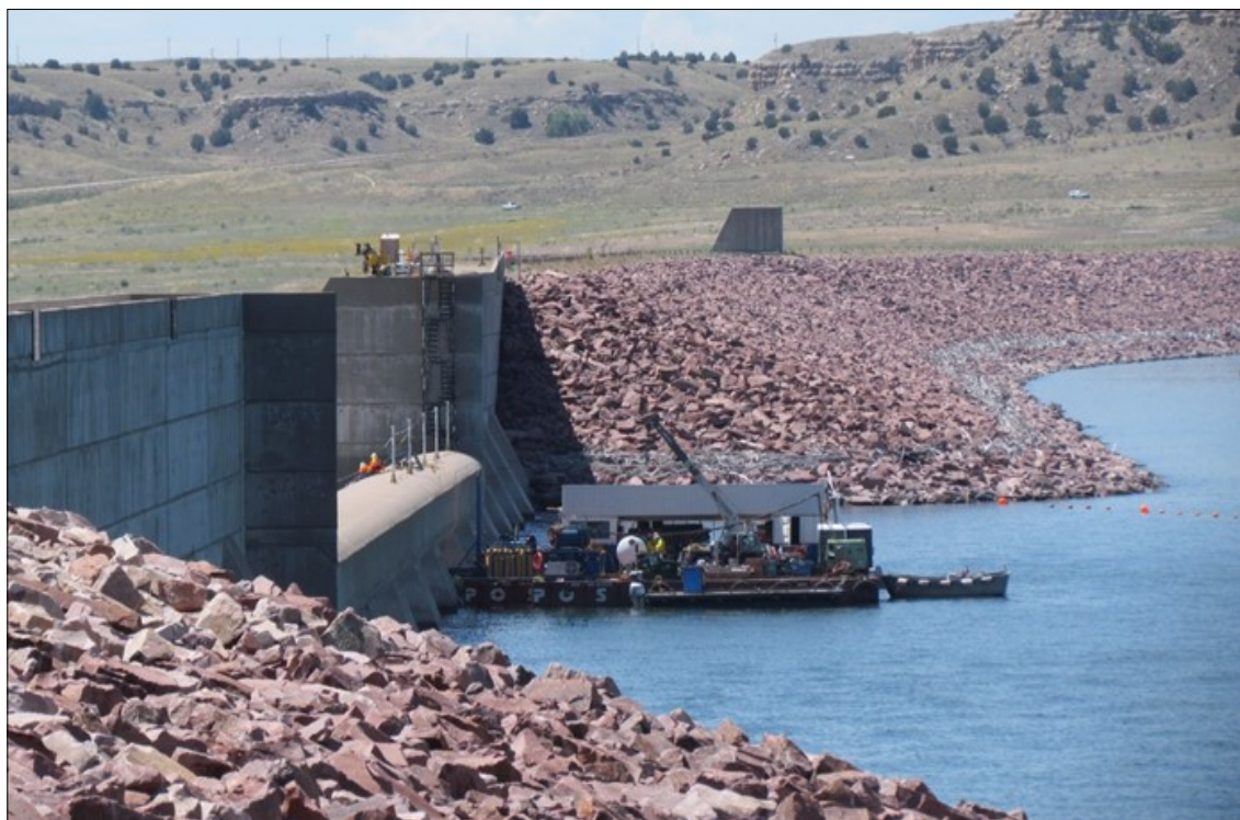
Restoration of the expansion joints between the concrete buttresses on Pueblo Dam began in 2019.
