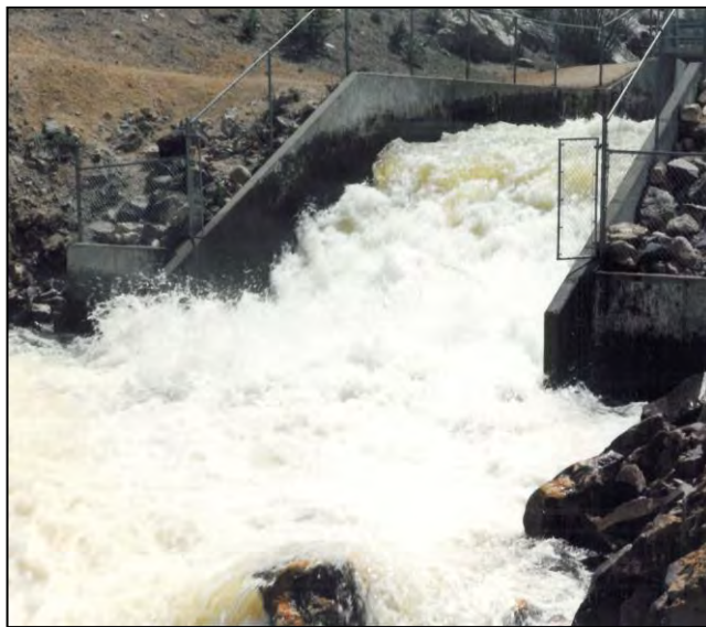
Boustead Tunnel Outlet
