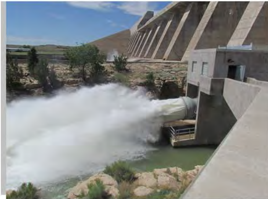
Pueblo Reservoir North Outlet
