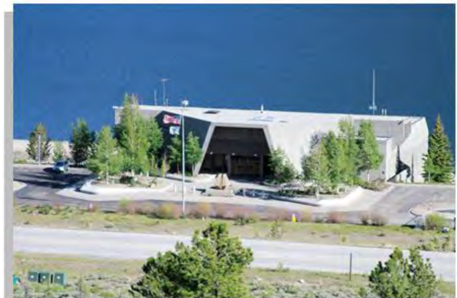
Mt. Elbert Power Plant
