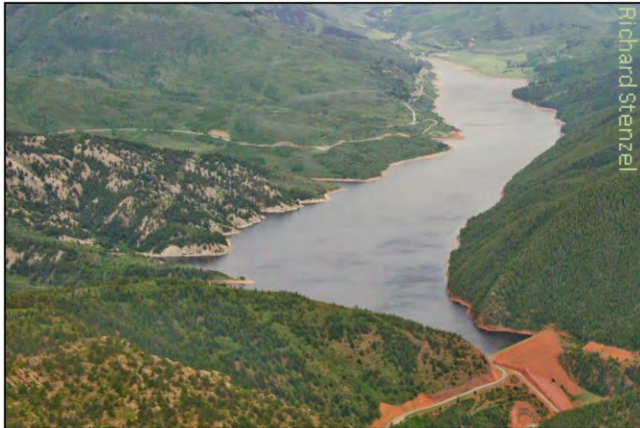
Ruedi Reservoir and Dam
