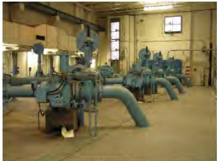
Water pumps for the Fountain Valley Conduit
