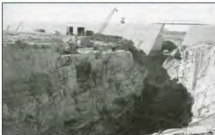
Pueblo Dam as it was being built in 1970. Shown is the buttress and spillway outlet and channel excavation.
