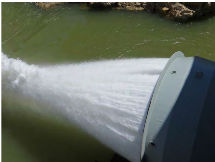
Pueblo Dam North Outlet
