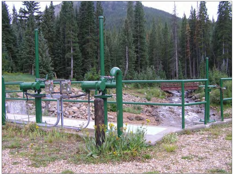
Intake of Boustead Tunnel on the Western Slope
