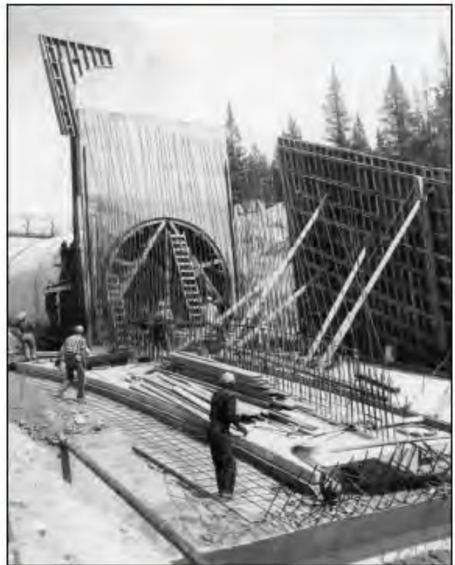
Construction at Ruedi Dam during the 1960s
