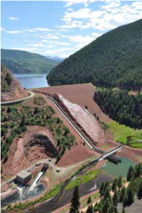
Ruedi Dam, spillway and hydroelectric plant
