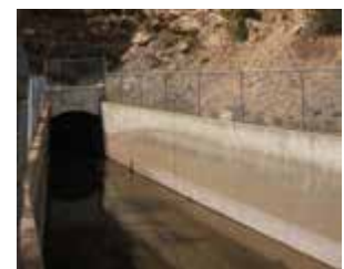
The Charles H. Boustead Tunnel conveys all the water collected in the North and South Side Collection Systems under the Continental Divide to Turquoise Lake.
