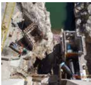
Construction on the Pueblo Dam North Outlet Works
