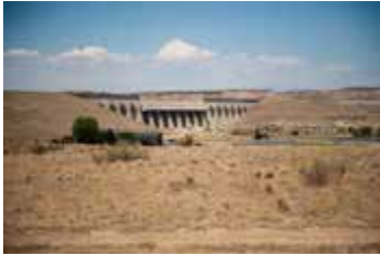
Pueblo Reservoir is located approximately 7 miles west of the City of Pueblo
