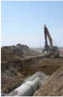
Reclamation sample picture of Conduit construction.
