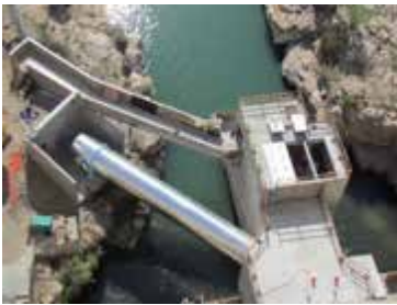
Southern Delivery System construction on the south outlet works of Pueblo Dam.
