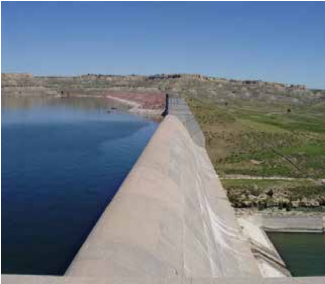
View of Pueblo Dam.
